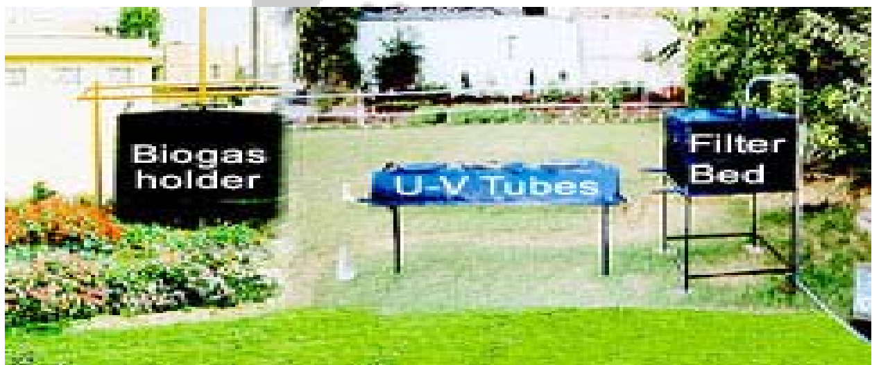
Human Excreta based biogas plant developed by Sulabh
